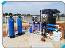
Filteration units can supply in mild steel (MS) with liners. Stainless Steel (SS 304 & SS 316) and fiber Reinforced Plastic (FRP).
